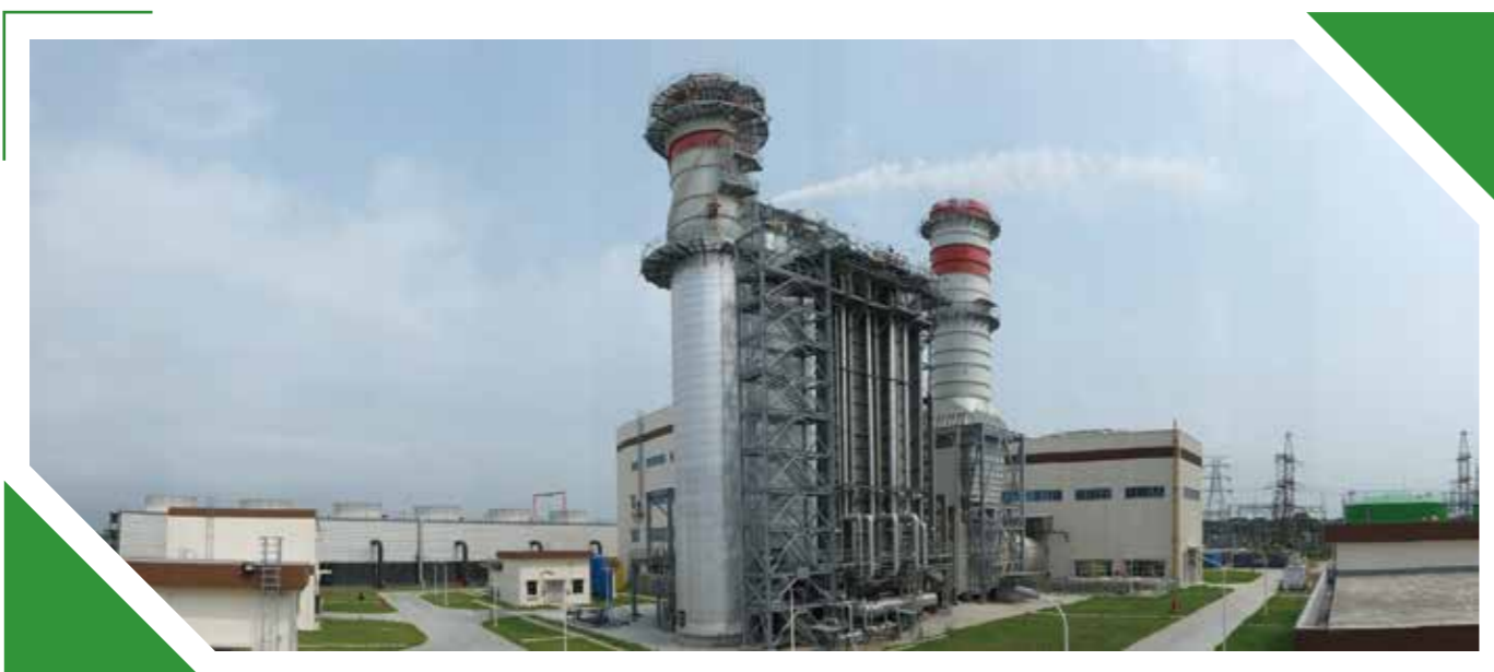
Construction of Ghorasal 300-450 MW Gas Based combined Cycle Power Plant Project by CNTIC
