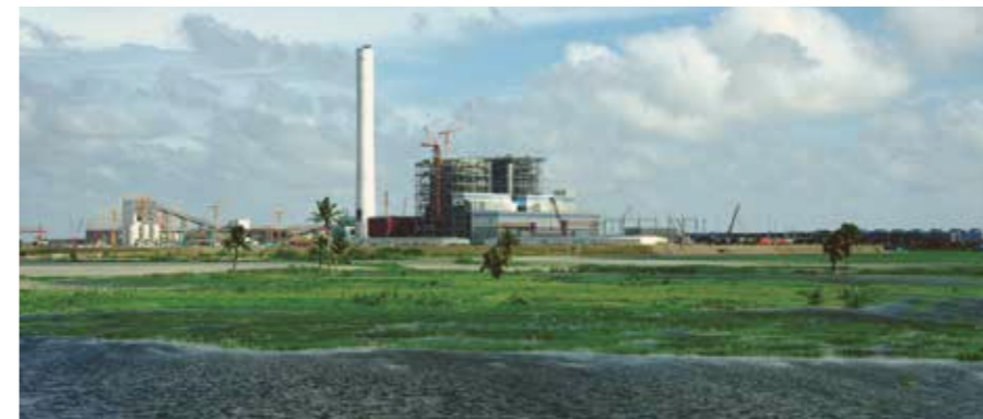
A distant view of the Payra thermal power plant
