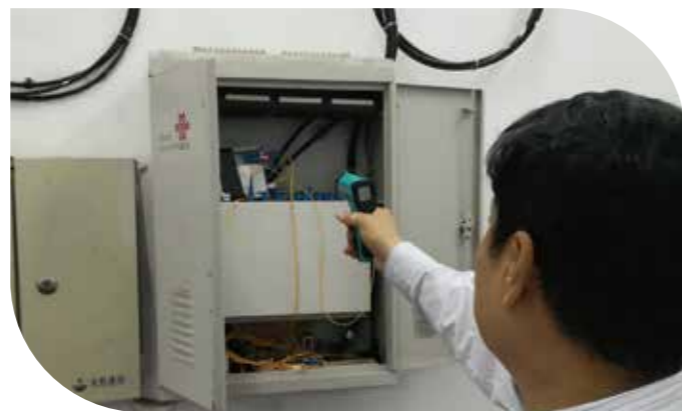
Work safety inspection at GENTRANS
