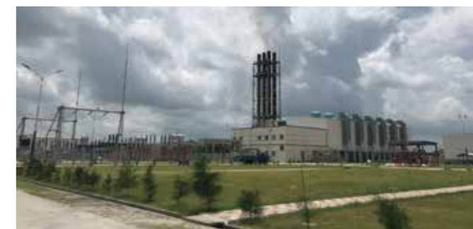
The greening of CMC's Madhumati 100 MW HFO Based Power Plant Project, Bangladesh
